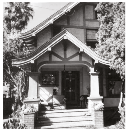
Soteria House in Santa Clara, California
